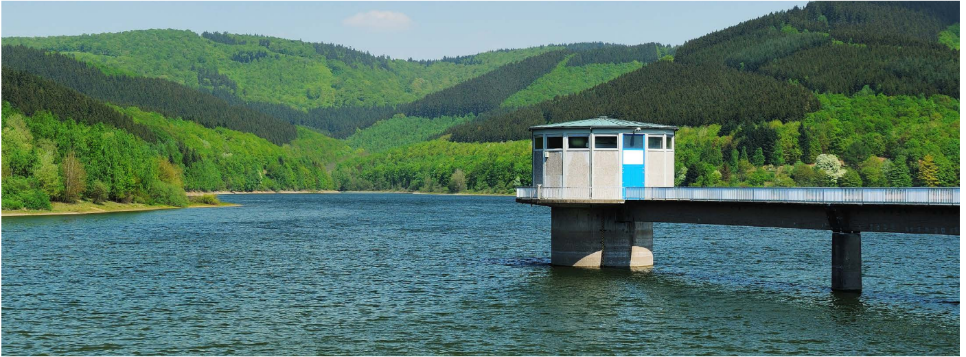
Figure 1: Drinking water reservoir.
